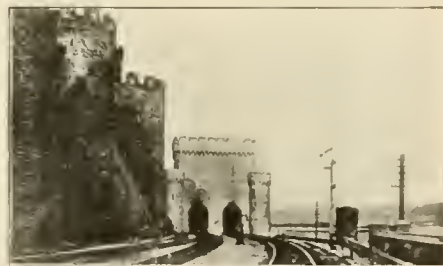
ENTRANCE TO CONWAY BRIDGE.
